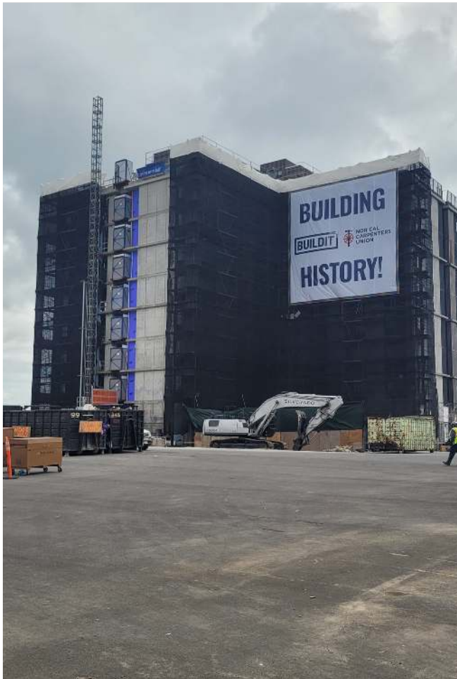
Oversized banner on a building under construction
